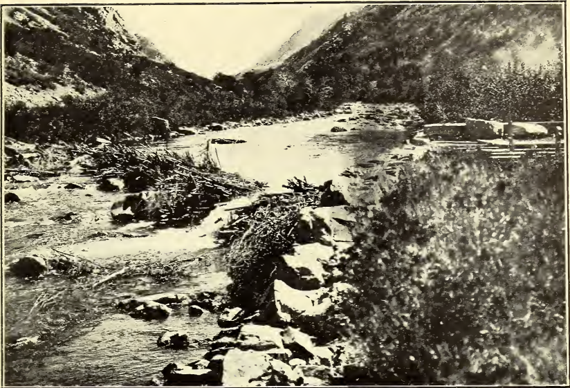
FIG. 1.—BRUSH DAM, WEBER RIVER, UTAH.
